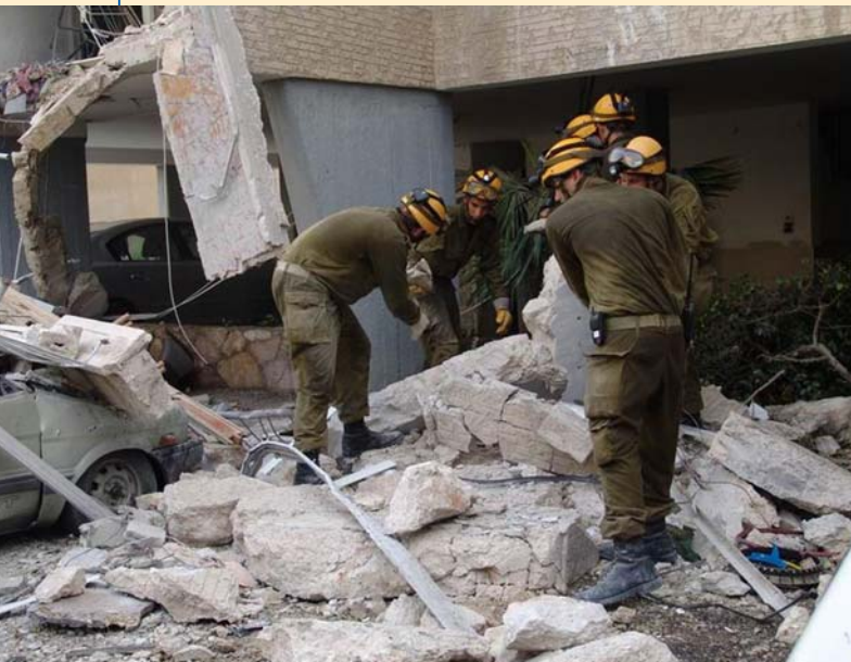
A view of some of the damage incurred in northern Israel
